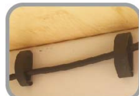
Cable Management Route cables neatly
